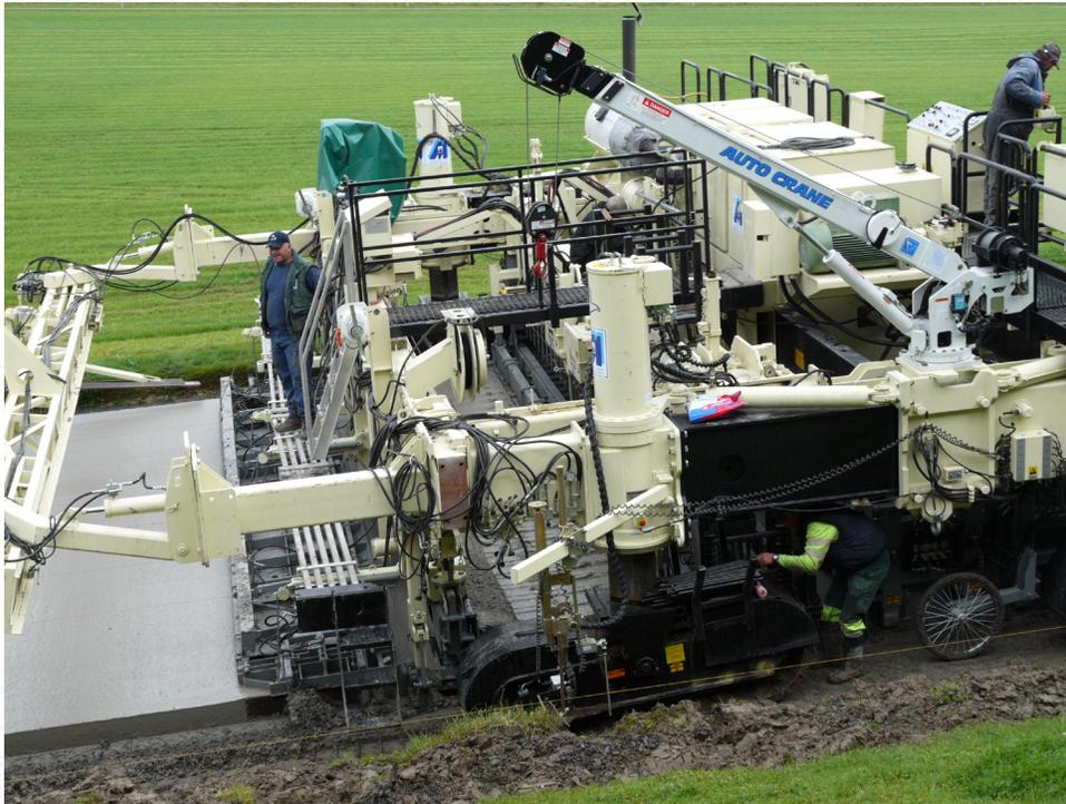
G&Z's patented mechanical Dowel Bar Inserter attachment accurately inserts dowels in plastic concrete behind the slipform paver confining pan. G&Z's unique combination of DBI confining pan, trailing sideforms and vibrating insertion forks help insure good consolidation and homogeneous concrete around the inserted dowel bars. This is accomplished while minimizing the disturbance to the surrounding concrete surface.
