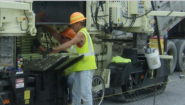
The CDBI is equipped with a dowel bundle support rack allowing dowel bars for several joints to be staged within reach of the operator for the loading of the chain feeder.
